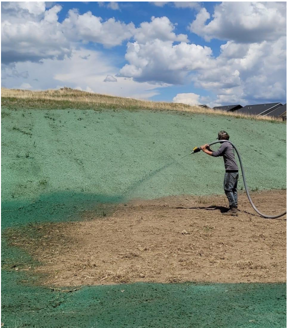
Hydroseed Installation Low
