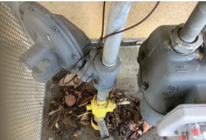
Gas feed with gas meter and GPR entering Art Center Building
