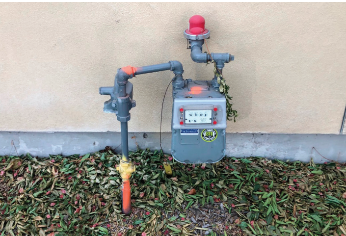
Gas feed with gas meter, GPR, and EQV entering AD/SS Building
