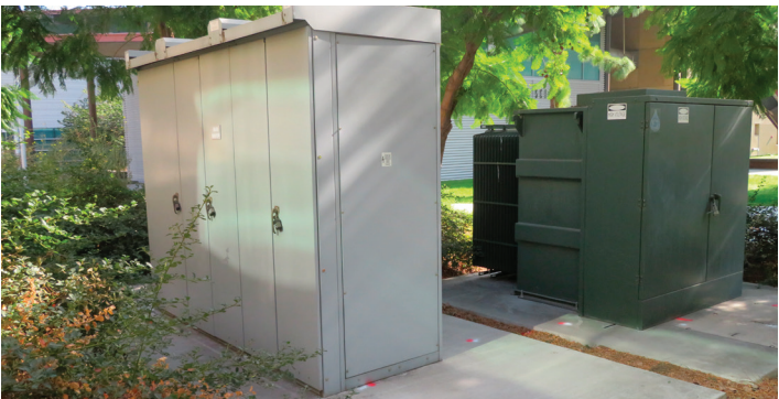
Physical Sciences Outdoor Padmount Transformer and Main Switchboard
