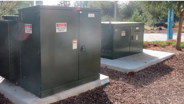
Selector Switch SS10 and Gymnasium Complex Outdoor Padmount Transformer
