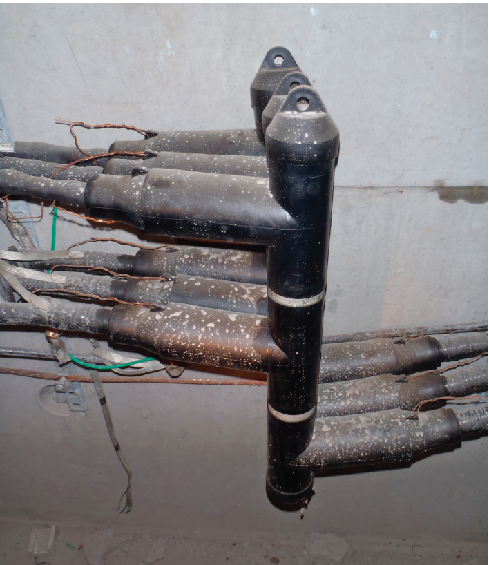
T-body Splice inside Electrical Manhole
