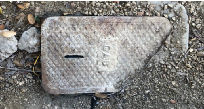
Gas vault outside Planetarium Building
