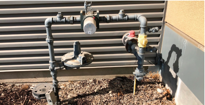
Gas feed with gas meter, GPR, and EQV entering Media Commons Building
