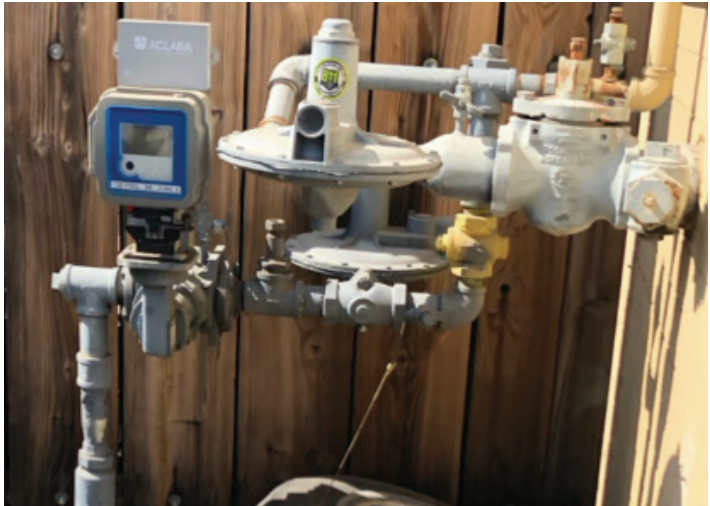
Gas feed with gas meter and GPR entering Applied Technologies Building
