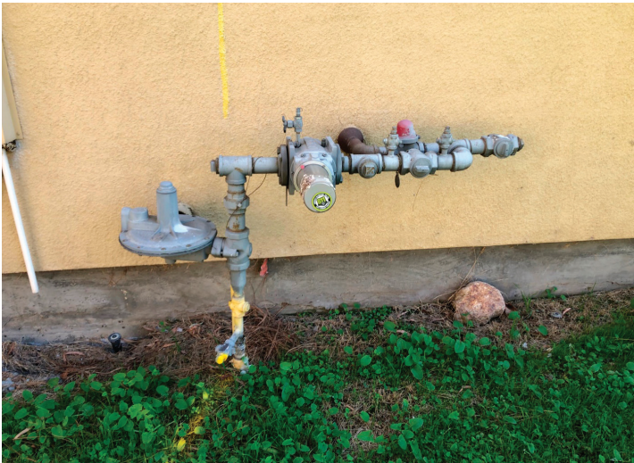
Gas feed with gas meter, GPR and EQV entering Library Building
