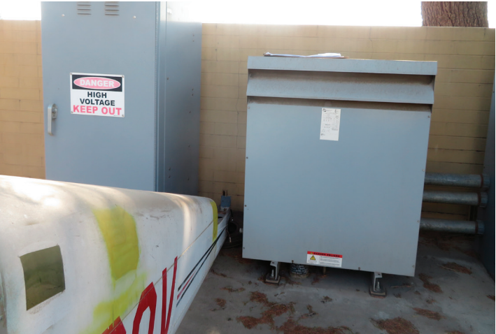
Technology Lab/Shop Load Interrupter Switch and Transformer
