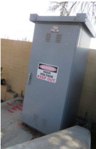
Technology Lab/Shop Load Interrupter Switch
