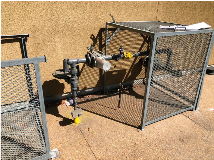
Gas feed with gas meter and GPR entering North Hall
