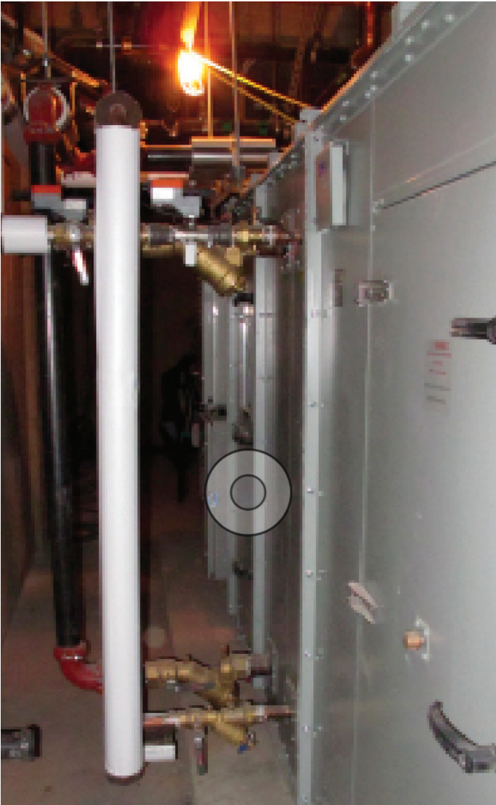
AHU Coil Connections at Business
