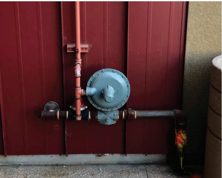
Gas feed with gas meter and GPR entering Physical Sciences Building
