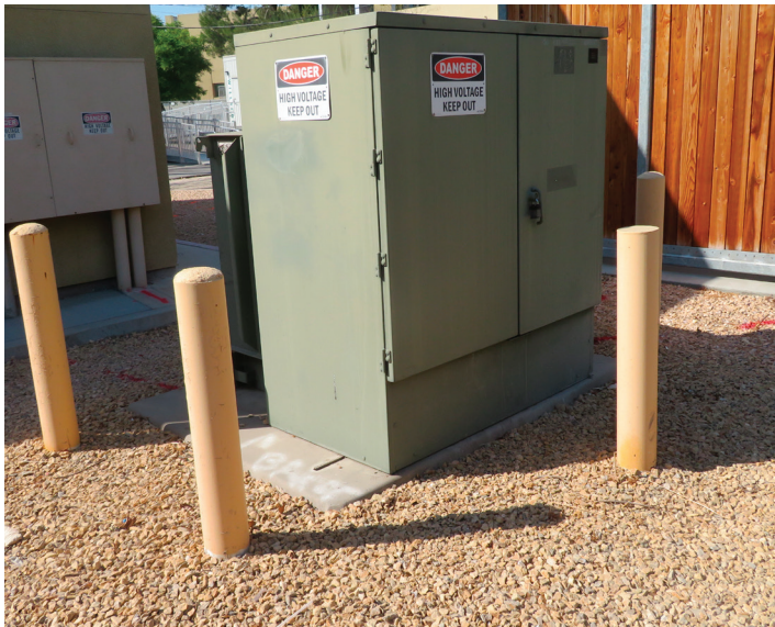
Outdoor Padmount Transformer at Media Comunnications Building
