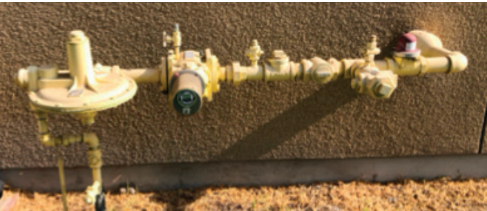
Gas feed with gas meter, GPR, and EQV entering Health and Life Sciences Building
