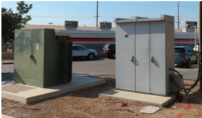
Computer Services Building Outdoor Padmount Transformer And Main Switchboard
