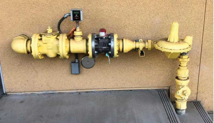
Gas feed with gas meter, GPR, and EQV entering Gymnasium
