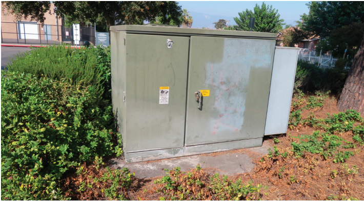
Child Development Center Outdoor Padmount Transformer
