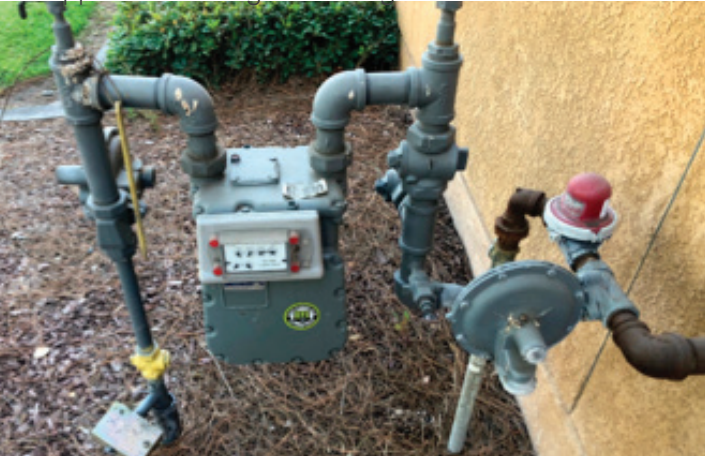
Gas feed with gas meter, GPR, and EQV entering Child Development Center
