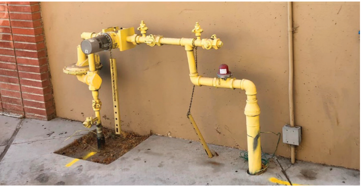
Gas feed with gas meter, GPR and EQV entering Business Building
