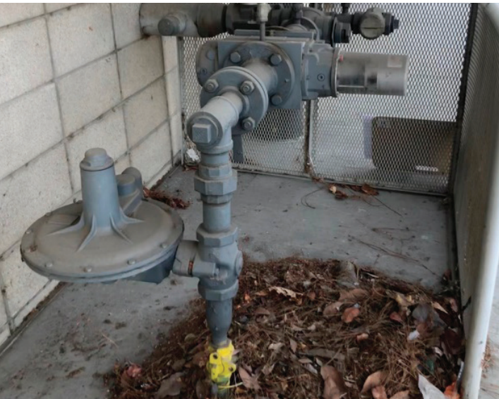
Gas feed with gas meter, GPR, and EQV entering Art Center Building
