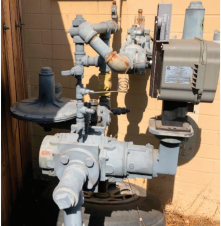
Gas feed with gas meter and GPR entering Applied Technologies Building
