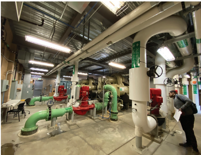
HHW Pumps at Central Plant
