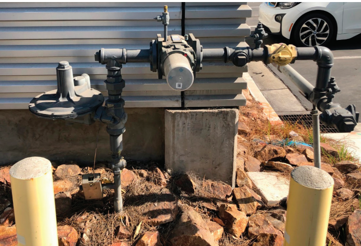
Gas feed with gas meter and GPR entering Power Station
