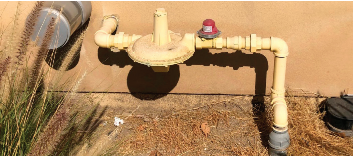
First gas feed with EQV and GPR entering Campus Center
