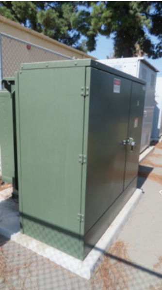
Technology Bungalow/ Classroom Outdoor Padmount Transformer
