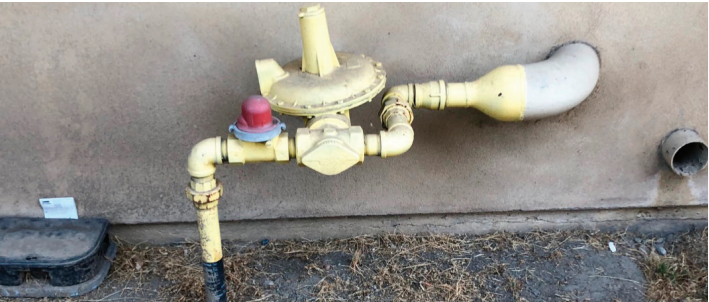
Second gas feed with EQV and GPR entering Campus Center
