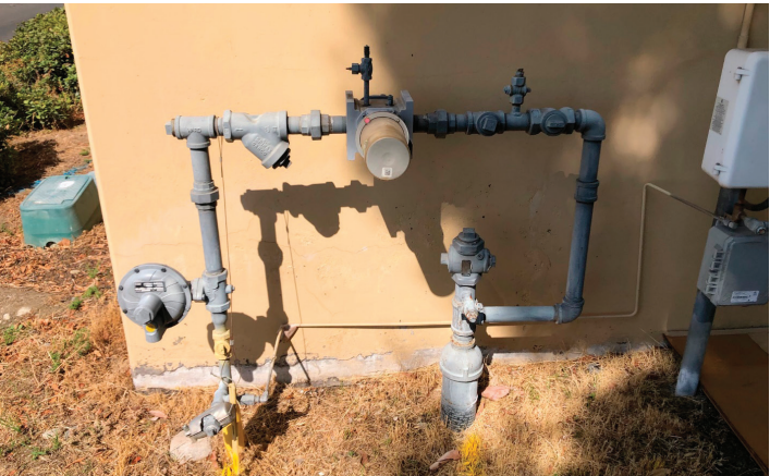
Gas feed with gas meter and GPR entering Liberal Arts Building
