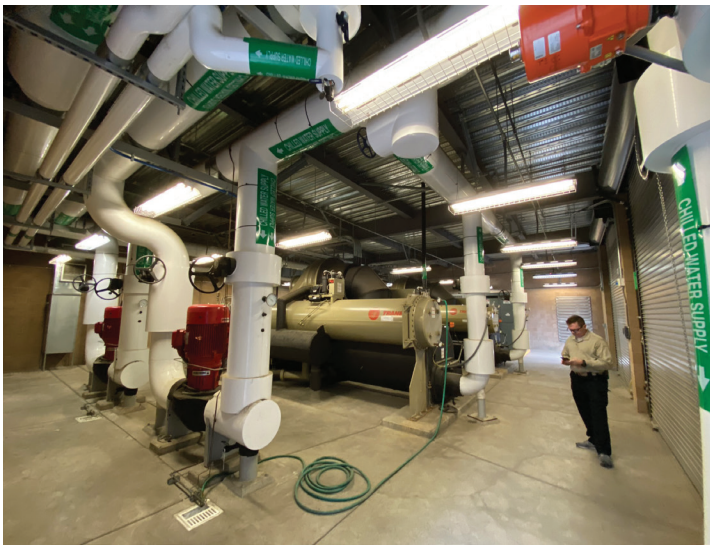
HHW Pumps and Chillers at Central Plant
