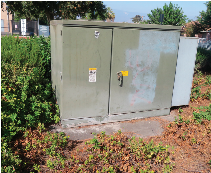
Outdoor Padmount Transformer at Media Comunnications Building
