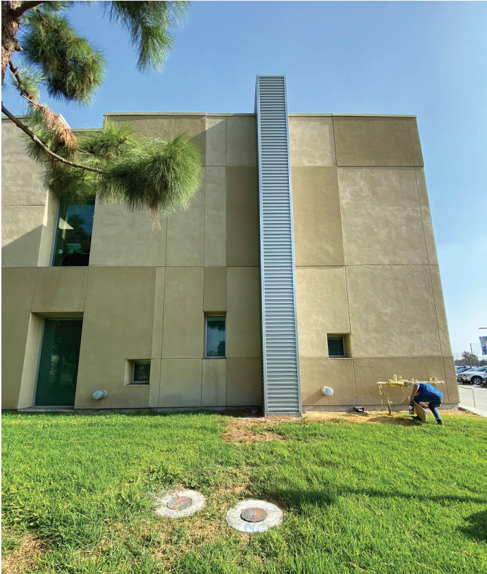
Chilled Water Pipe Chase
