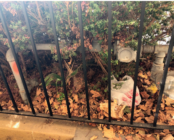
Gas feed with gas meter and GPR entering Auditorium Building valve.
