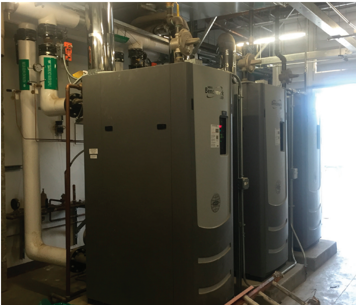
Condensing Boilers at Gym
