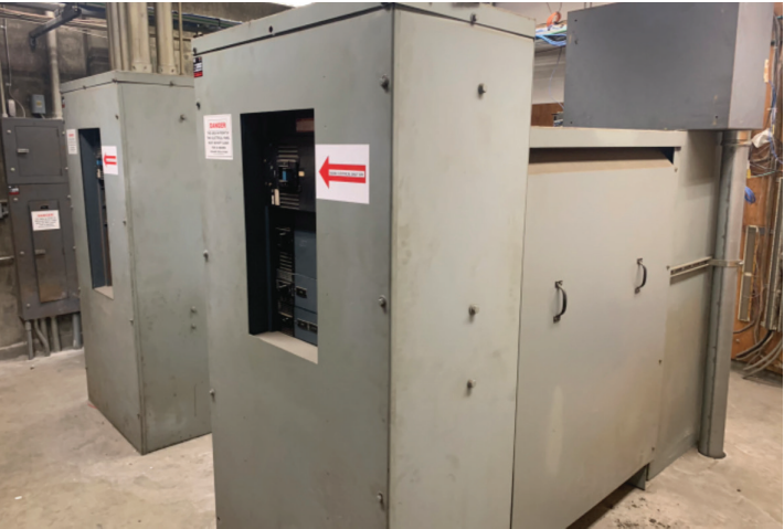
Liberal Arts Building Load Interrupter Switch and Transformer
