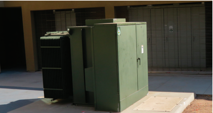
North Hall Outdoor Padmount Transformer and Main Switchboard
