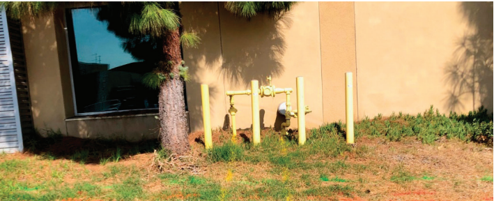
Gas meter and GPR assembly outside southern side of the Campus Center
