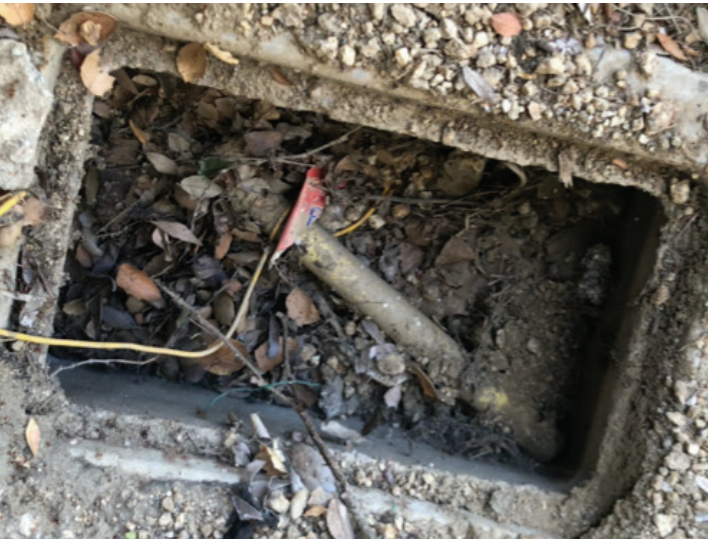
Gas feed entering Planetarium
